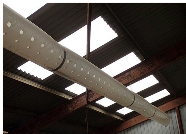
Positive pressure air tubes can be used to improve the ventilation in existing sheds.
